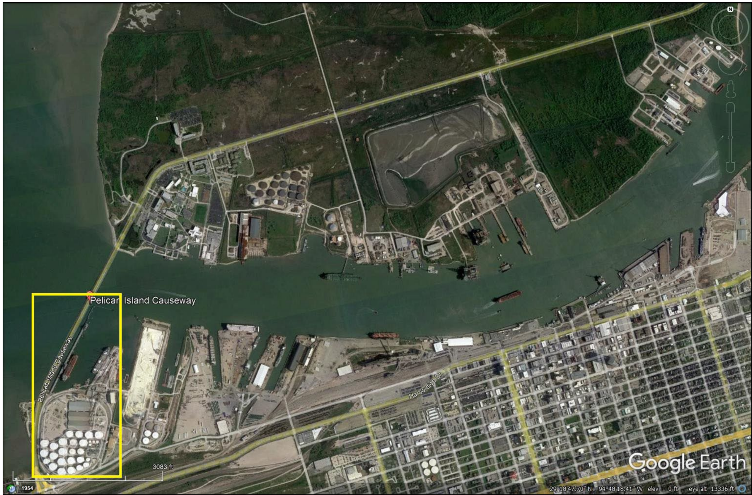
Figure 5 - 2022 Aerial Photography showing Docks Built Since 2017 Authorized Plan
